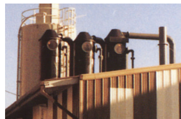
Tri-NO x scrubber through-the-roof installation.
